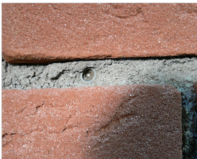
Facamax spanningsvrije bevestiging gereed.
